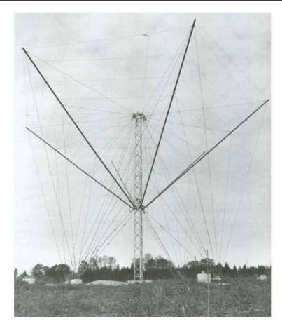
The SPIRA-CONE uses a four-arm conical logarithmic spiral with interleaved wire elements and does not require a groundscreen.
