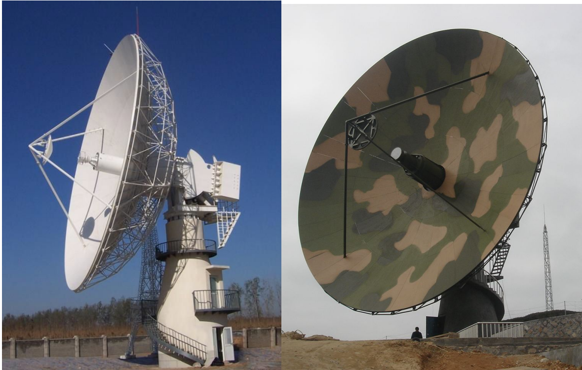
Super 16m antenna ( Rotation type)
