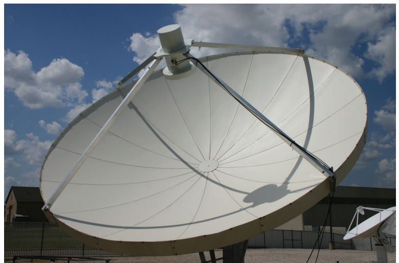
Typical Installations of GRBF-100 and GRBF-200-CLA Feeds
