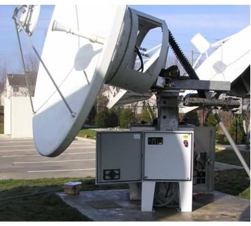
Enjoy the High resolution and accuracy of resolvers as position sensors on antennas equipped with Single-Speed, 3-phase AC Motors. Allows the use of the RC2500 with virtually any antenna system.
